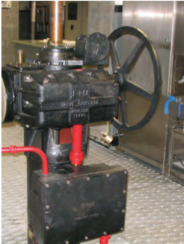
Current M2CP units evolved from proven technology—as shown by this EIM actuator, still operating after more than 50 years at a water distribution and storage system in New York City.
