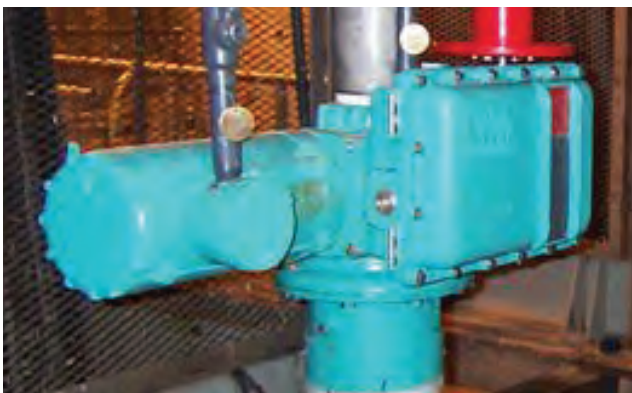
EIM AquaNaught variant of the M2CP actuators can withstand extended submersion.
